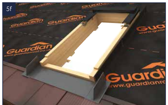
5f Roof windows should be installed with a compatible slate flashing kit.
