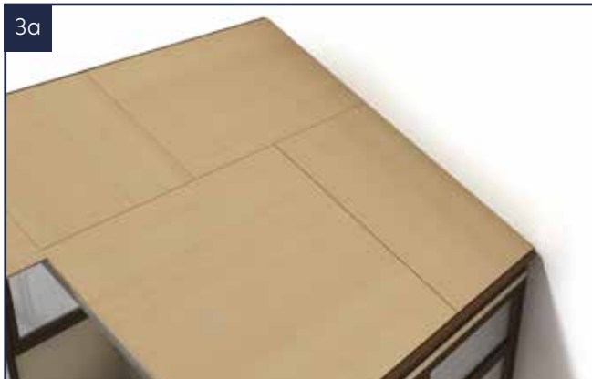
Fix plywood sheets to rafters as per roof schedule.
