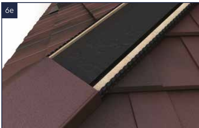
Ensure the ventilation strip is fixed to the timbers.
