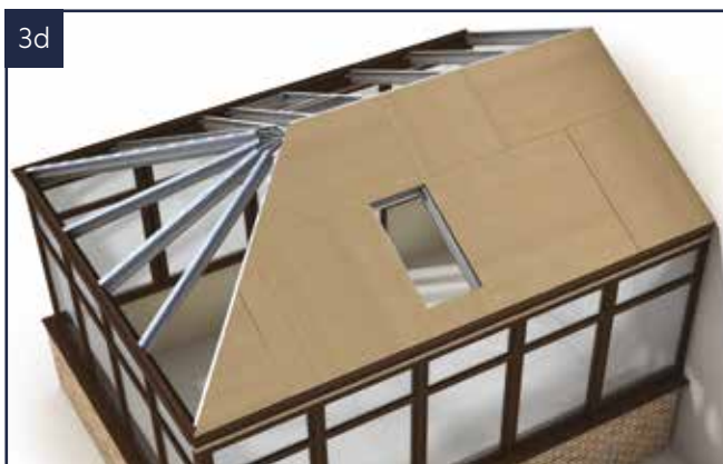
Finish the first side then continue around the whole roof.
