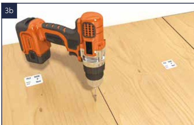
Plywood sheets to be fixed at no more than 200 mm centres using 4.8 x 38 mm self-tapping fasteners (drill pilot holes).
