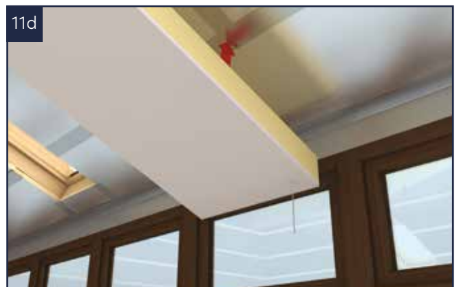
11d Cut and mitre 72 mm insulated foil backed plasterboard, fix into position at no more than 50 mm in from the corner and at no more than 200 mm centres with fixings supplied.
