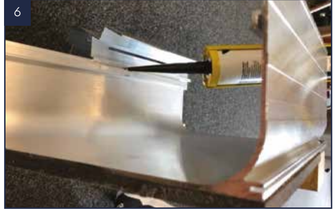
6 If not already sealed, run a bead of silicone along the top edge of the joint between the eaves and boxgutter.
