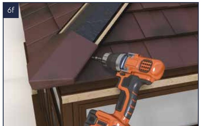
Fit endcaps and fix on both sides. Use touch up kit provided to hide screw heads.
