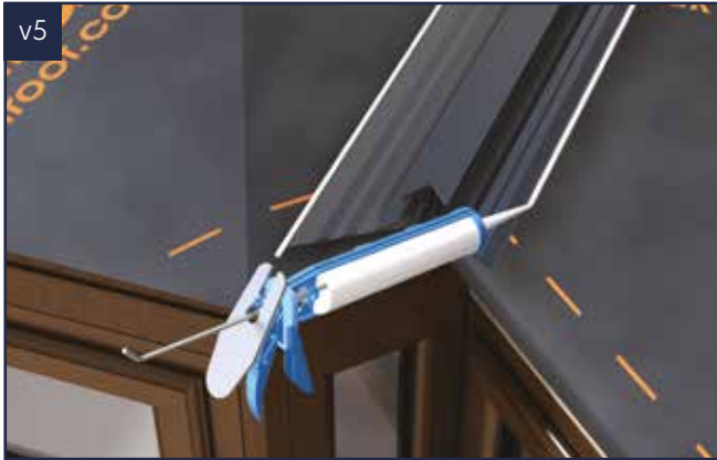
Run a bead of silicone down both edges of the valley to dam against the membrane.
