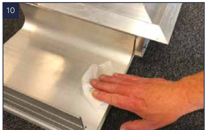
10 Ensure aluminium gutter is clean dry and grease free.
