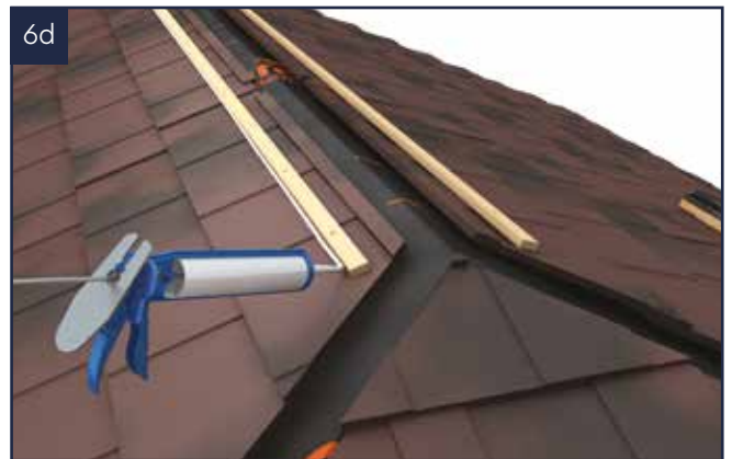
Use low modulus silicone between the front edge of the roof batten and tile.
