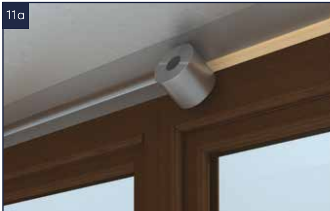
11a 75 mm insulated foil tape should be used around the top of the window frames to cover any exposed timber.
